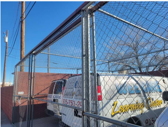
Nearby day care — insufficient overhead coverage, not secure enough
